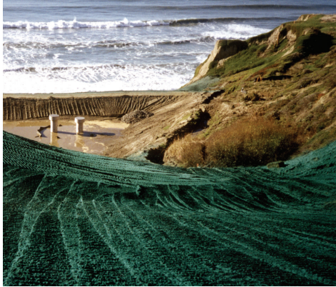
Less expensive than extended term blankets, and less soil preparation is required
